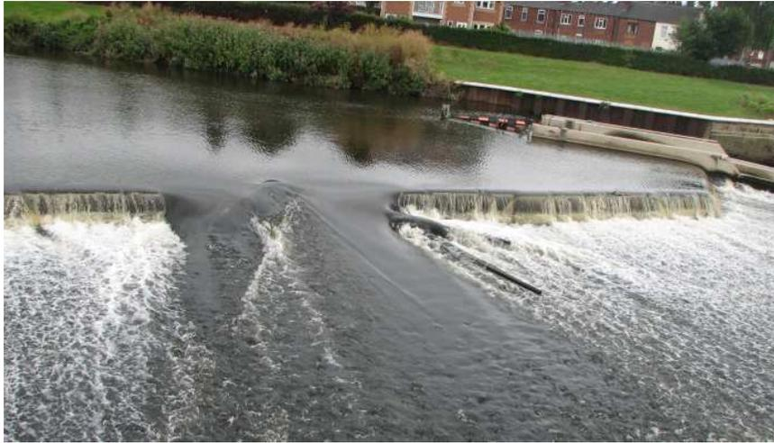
**Broken weir board in centre of weir**
