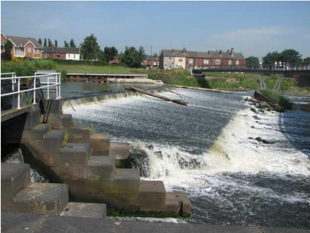
**Figure 1a: View from the sluices across the weir apron**
