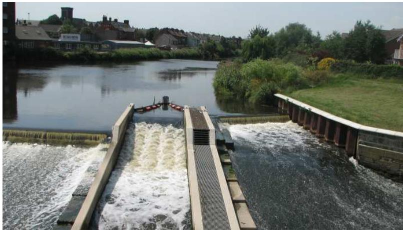
**Figure12:Larinier pass on bank opposite proposed turbine location.**
